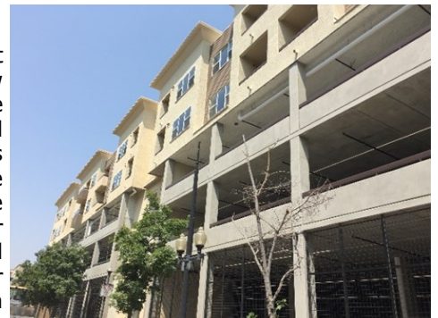
Pictured: Bridges north building
