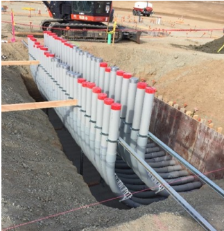
Pictured: Sky Ranch Middle School hydroponic piping
